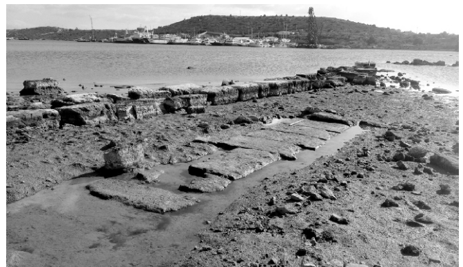
Fig. 4. Salamis. Part of the foundation course of a strong well-built structure of the Late Classical-Roman period, close to a later mole constructed with ancient stone material, on the north side of the Bay of Ambelaki (photo Chr. Marabea).
